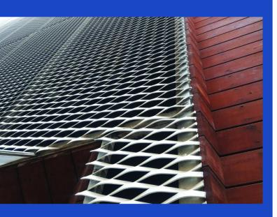
Expanded metal or stretch metal refers to metal plates (iron, aluminium, steel, etc.), which are stilled and stretched with a specific technique while passing through the manufacturing process. Stretch metal panels with different thicknesses and customized colours can be implemented based on the powder or electrostatic method, and cutting through a CNC machine.
